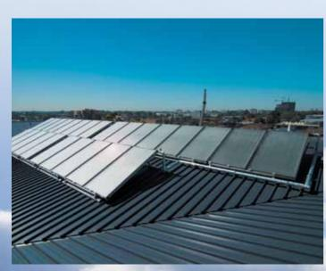
Closed loop, split solar is Rheem NZ's Premier Solar system which is designed for top performance in our environment, even when it is frosty or the water quality is poor. This revolutionary system combines Rheem NZ's high efficiency T200 collector with a heat exchange cylinder to heat and store 270 litres of water.
