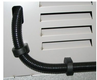
Step 11 fix conduit clamp to heat pump module and locate cable set conduit
