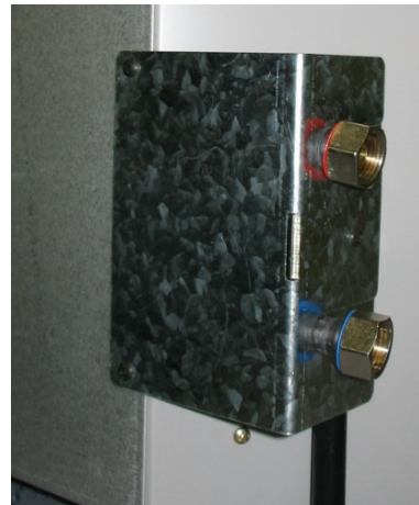
Step 10 fix rear access panel and hose bracket assembly to heat pump module
