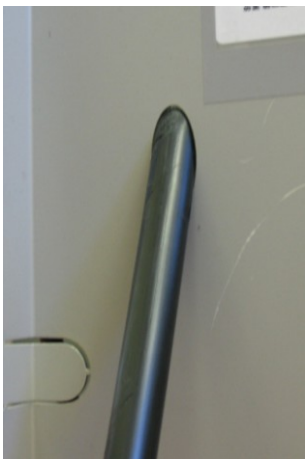
feed hose through penetration
