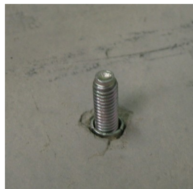
Step 14 drill holes in slab or solid base and insert dynabolts
