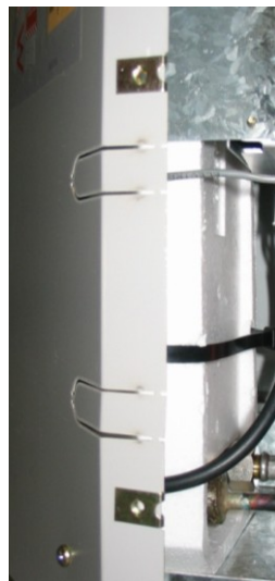
Step 9 clip speed fasteners to the heat pump module casing
