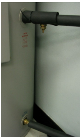
Step 22 connect insulated heat pump circuit pipe work to heat pump module and heat pump storage tank
