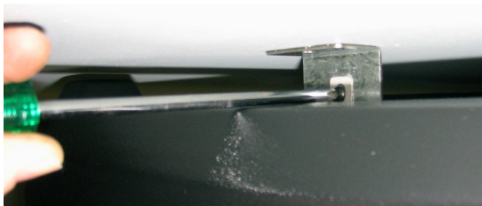
Step 18 fix wall bracket tab to wall bracket
