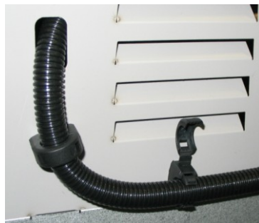
Step 11 fix conduit clamp to heat pump module and locate cable set conduit
