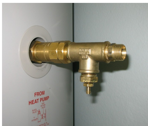
Step 20 connect non return valve and air bleed valve assembly
