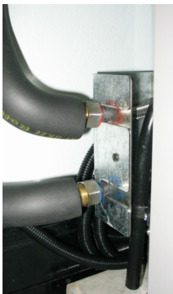
Step 22 connect insulated heat pump circuit pipe work to heat pump module and heat pump storage tank
