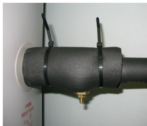
insulate non return valve and air bleed valve assembly
