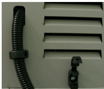
Step 11 fix conduit clamp to heat pump module and locate cable set conduit
