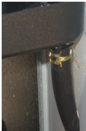
Step 4 secure hose to the spigot
