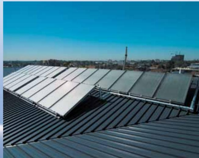
Closed loop, split solar is Rheem NZ's Premier Solar system which is designed for top performance in our environment, even when it is frosty or the water quality is poor. This revolutionary system combines Rheem NZ's high efficiency T200 collector with a heat exchange cylinder to heat and store 270 litres of water.
